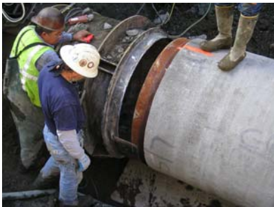
Construction workers joining 2 sections of 48" concrete cylinder pipe
